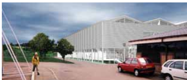
Chester-le-Street cricket academy. © David Morley Architects
